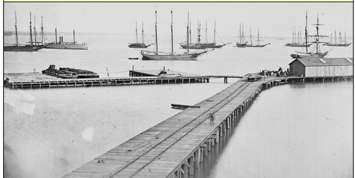
The photo above shows the rebuilt magazine storehouse, placed on a wharf extending far out into the James River at a safe enough distance that there would be no repeat of the Aug. 9 th disaster. Note the railroad tracks leading out to the storehouse, allowing ordnance to be quickly loaded or unloaded.
